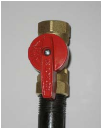
Gas Dryer Shut-Off.
